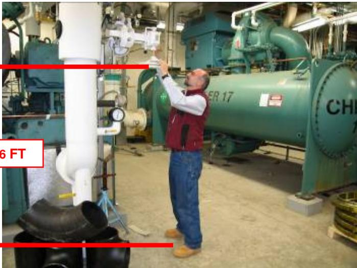
Relocated chiller is 500 tons – allowing for the smallest chiller to remain operating to maximize the free cooling. 3 pass configuration shown – opposite end connections
